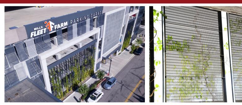
Starfleet rain screens are ideal for parking structures where creativity can be explored. Custom designed aluminum perforations create a unique aesthetic to plain garages, while allowing the required light and airflow to go through.
