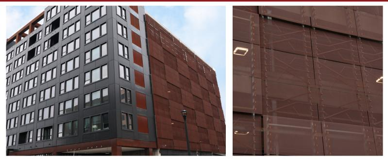
These cost effective, vertical support panels are formed to created rigidity and strength to meet code for parking structures and building facades. Aluminum perforated metal patterns come in a variety of shapes and sizes for a truly unique facade.
