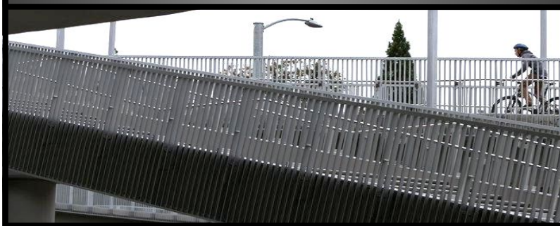
Vega Picket Guardrail
